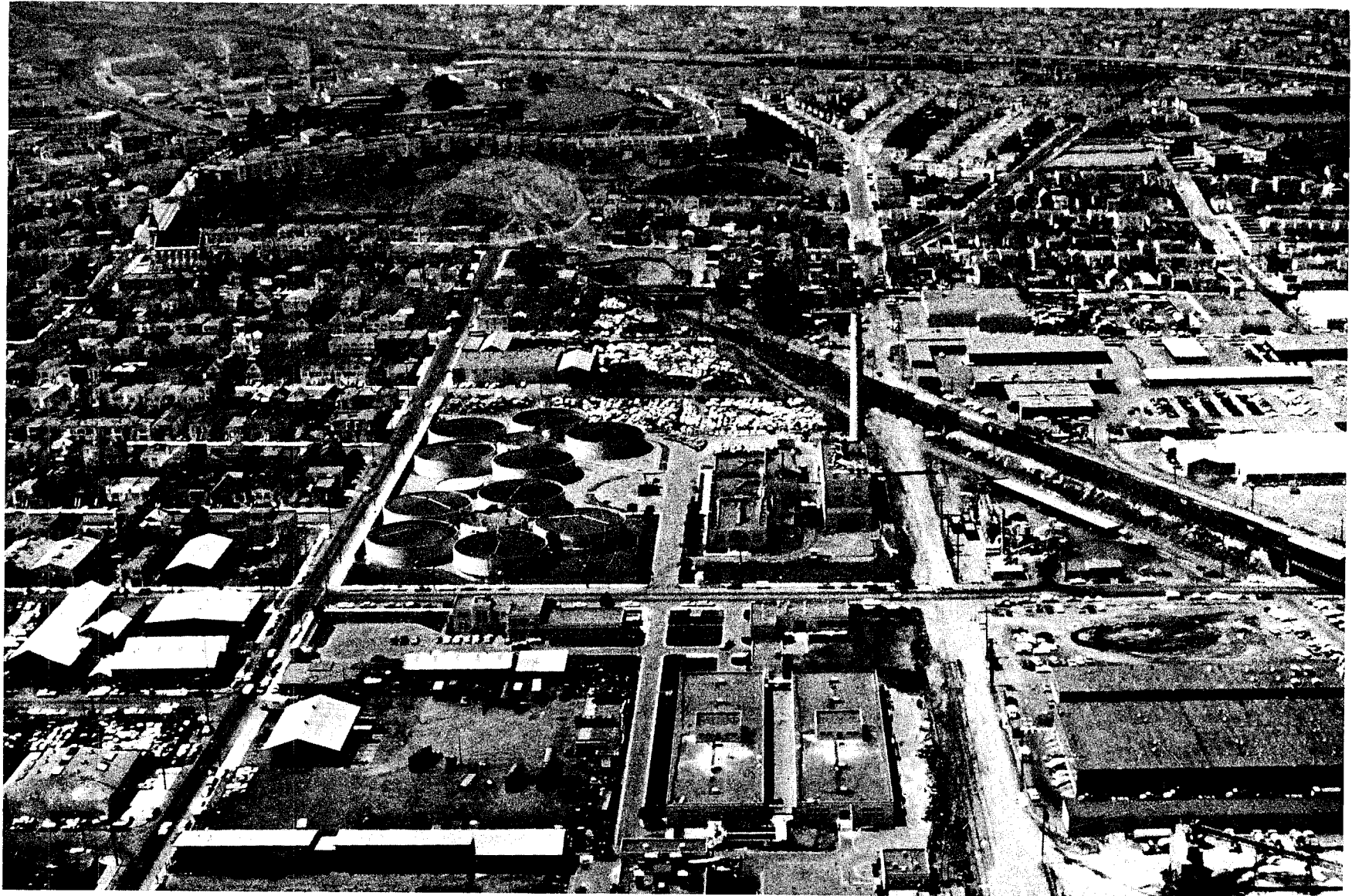
FIGURE II-6 SOUTHEAST WATER POLLUTION CONTROL PLANT
